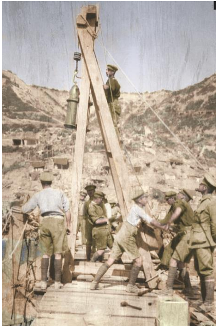
Constructing Watson's Pier
