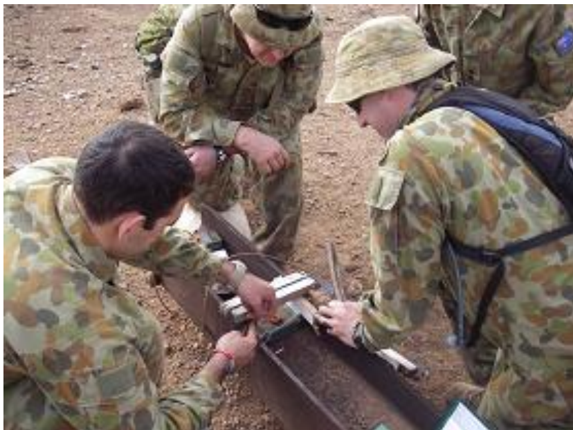
Sappers preparing explosive charges on a steel "I" beam
