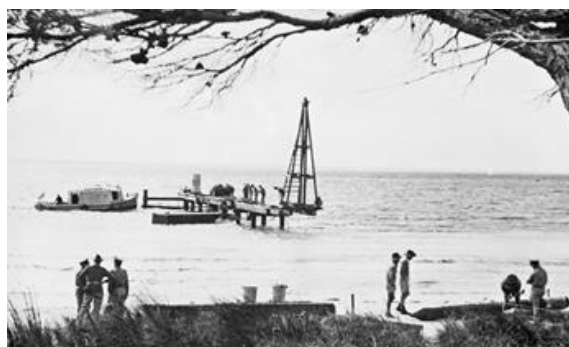
7 Army Troops Company constructing Sulphur Bay Jetty in March 1943.
