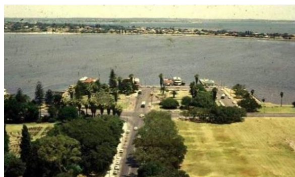
Barrack St Jetty & South Perth
